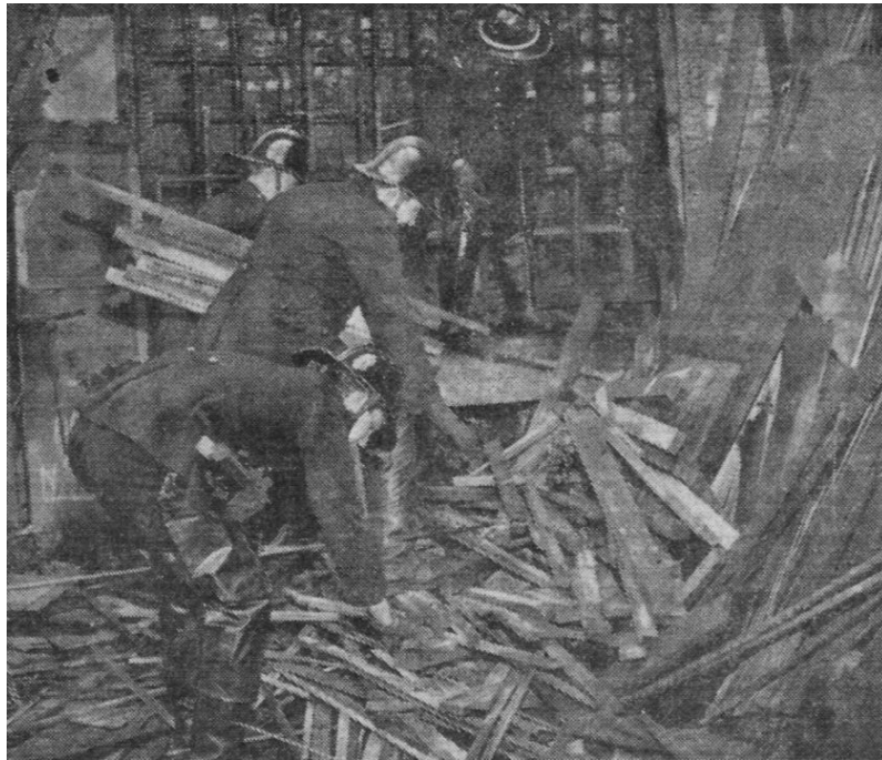
Firemen clear up the debris in the gutted workshop.
