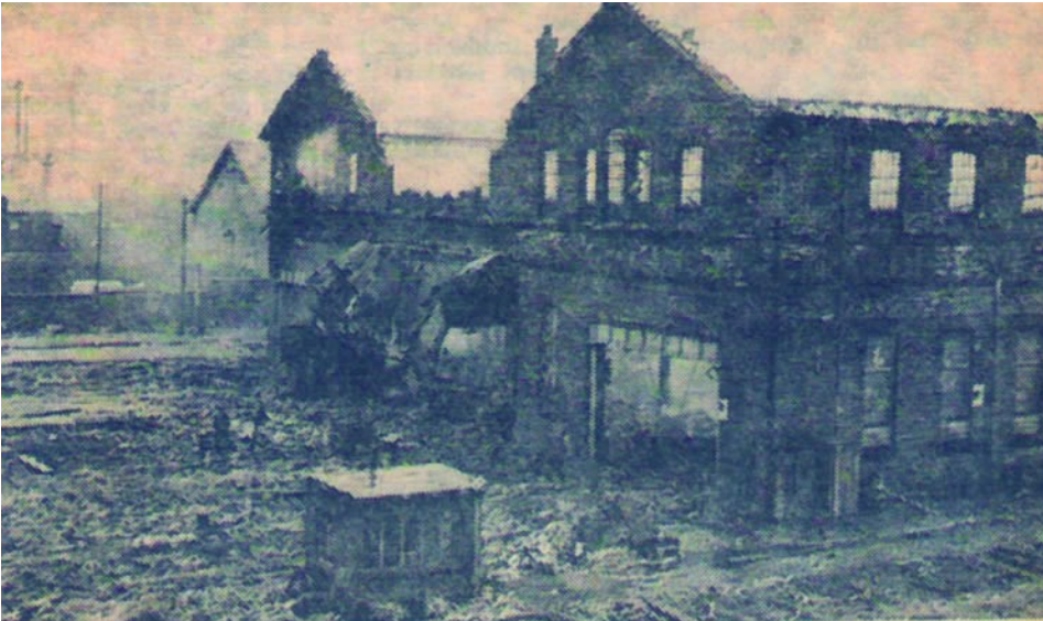
The gutted shell of the depot today, with smoke still rising from piles of debris
