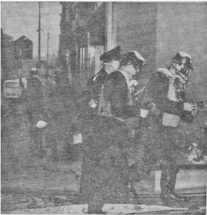
Firemen wear breathing apparatus to beat the smoke in the Sheffield fashion store of Price and Co. (Broomhill) Ltd. A showroom floor was damaged.
