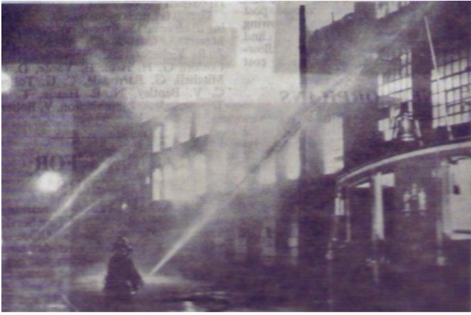
Weakened walls collapse into fire area
